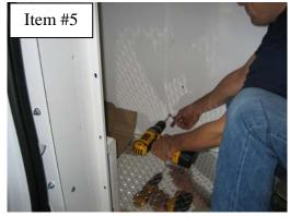
Remove screws holding the center divider together where 3<sup>rd</sup>
